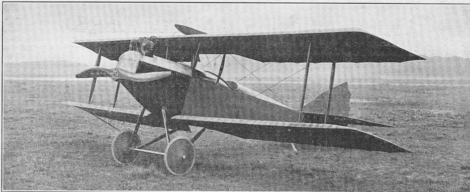
The Snyder-Macready light plane, fitted with an Indian Chief motorcycle engine. This ship, built in 1920-21 and flown then by Lieut. J. A. Macready, is a good example of scale-reducing a conventional airplane to a light plane
